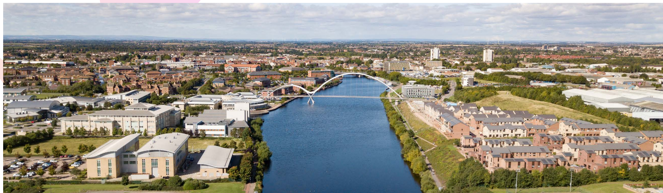
The Infinity Bridge connecting the town with the university
