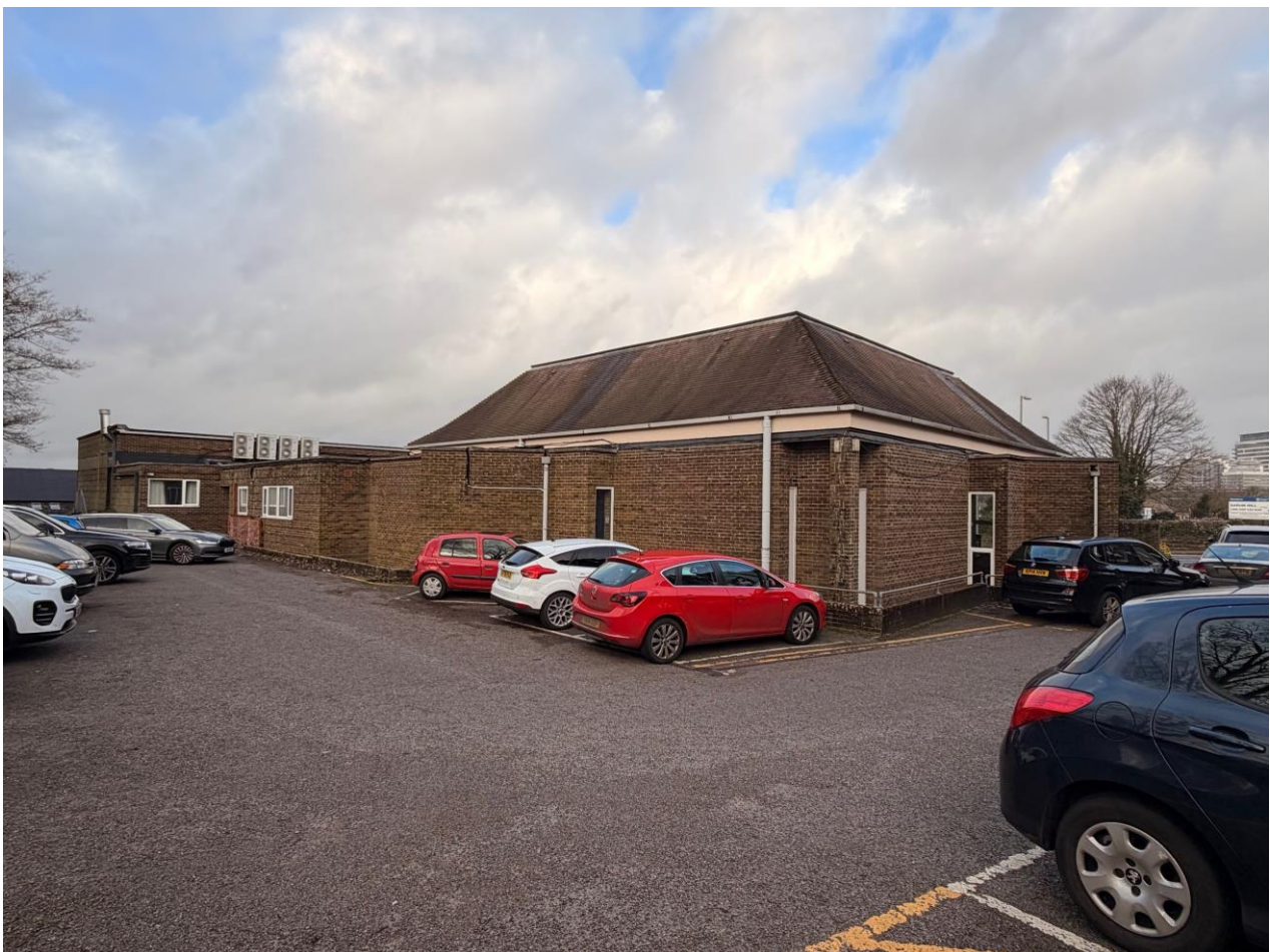
View of the property's rear elevation looking north
